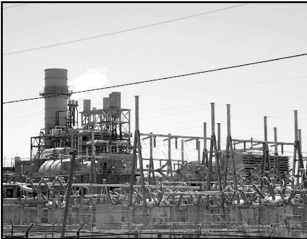
Los Medanos power plant located in Pittsburg, California was built under a PLA. Photograph by Joshua Mann, California Research Bureau.
