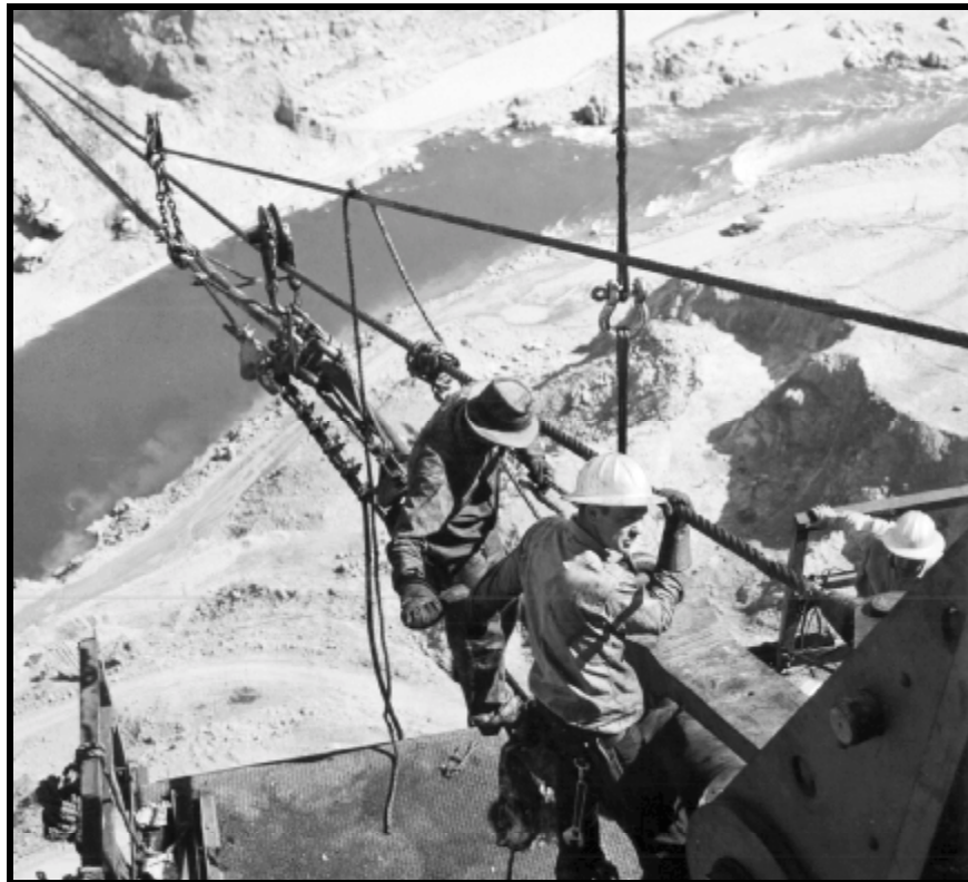
Shasta Dam, May 8, 1940. The head tower and riggers at the top of the 460 foot cable way. The cable was 3" in diameter and weighed 22 pounds per linear foot. Photograph by R.A. Midthun, courtesy of U.S. Bureau of Reclamation.
