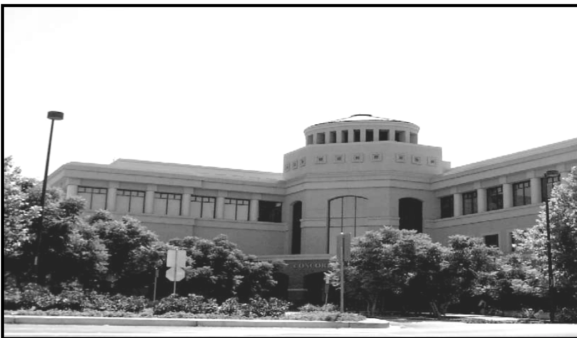
Police station in Concord, California constructed under a PLA. Photograph by Joshua Mann, California Research Bureau.
