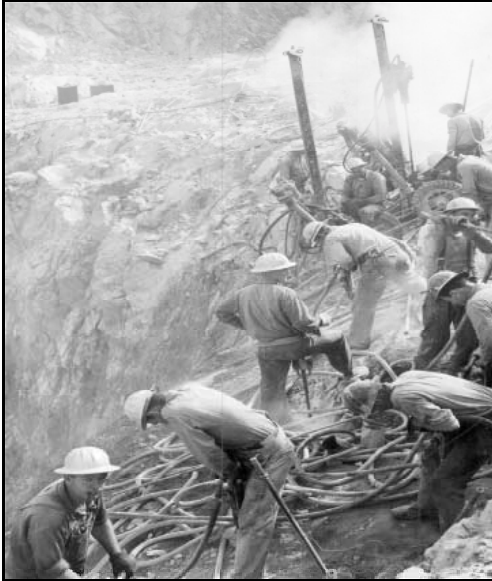
Shasta Dam, May 6, 1940. Battery of wagon drills and jackhammers making blasts in the right abutment at about 650 feet elevation. Photograph by R. A. Midthun, courtesy of U.S. Bureau of Reclamation.
